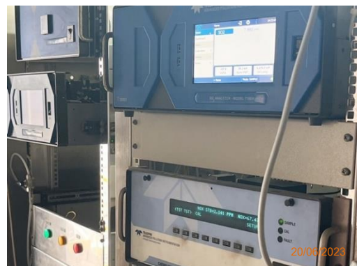
CEMs Recovery Boiler
